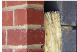
Cavity wall insulation
