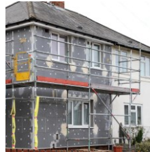
External wall insulation
