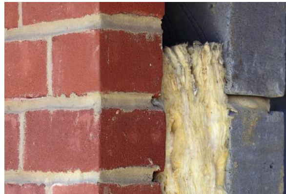
Cavity wall insulation
