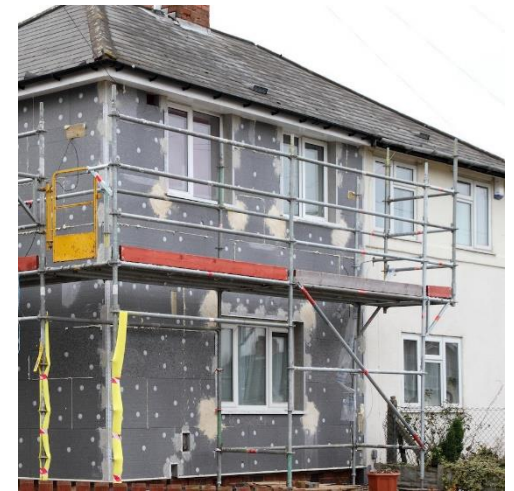
External wall insulation
